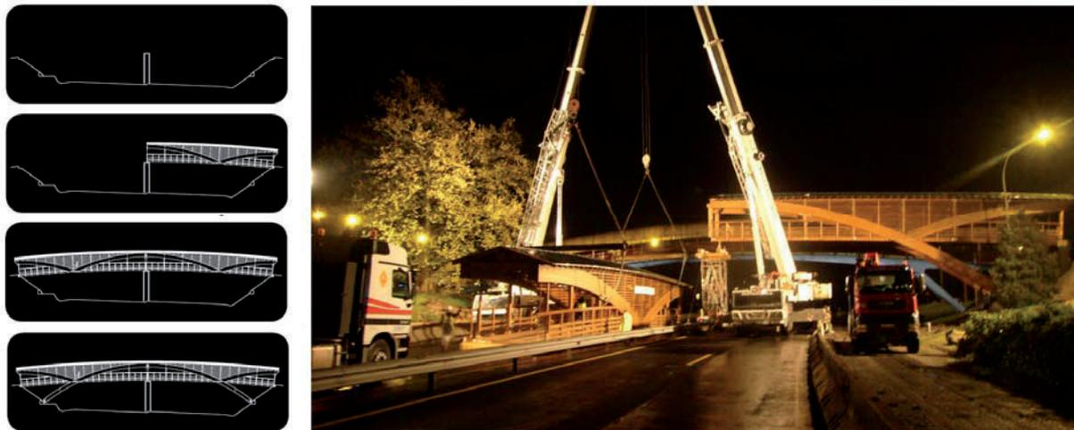
Fig. 2. Assembly sequence of the footbridge
