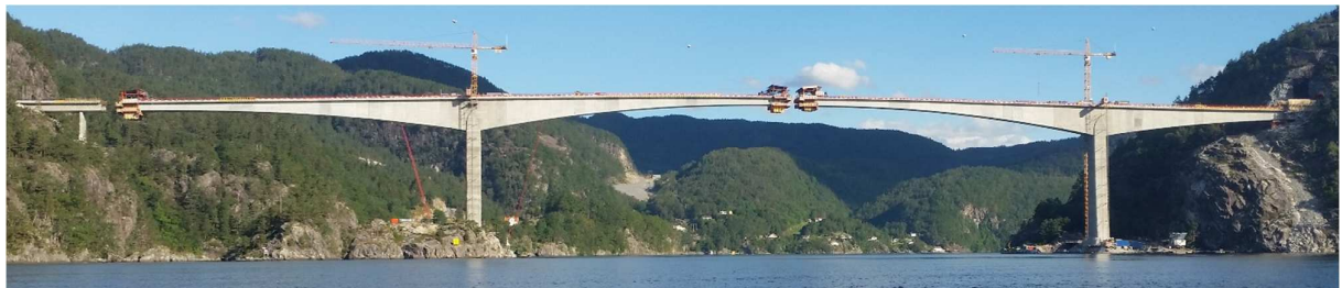
Figure 1. Sandsfjord Bridge from the south side, just before the bridge is continuous (axis 1 to the right)
