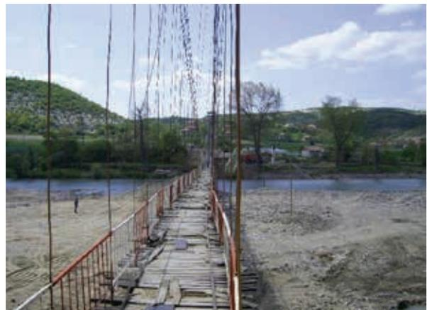
Figure 1: Bridge superstructure before the reconstruction
