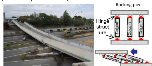
Figure 1. Damage of rocking piers
