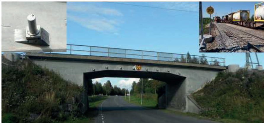
Fig 1. Haparanda bridge. The left insert shows one of eight post-stressed bars installed in holes drilled through the slab. The right insert shows traffic on the two tracks on the top of bridge.
