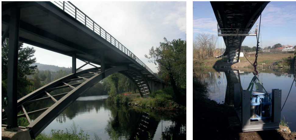
Fig. 1: (a) General view of footbridge at Parque da Rabada, Portugal; (b) Installation of TMD
