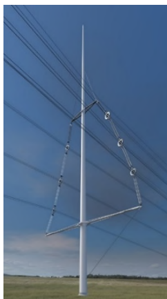
Figure 1 : The new concept of high voltage overhead line between Avelin and Gavrelle (France)
