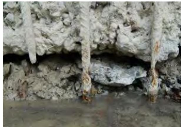
Figure 1. Typical loss of rebar cross-section due to advanced corrosion at the earth-covered rear side of an angular retaining wall [3]
