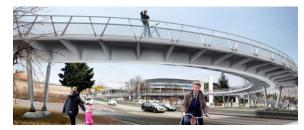
The new bridge is conceived to minimise travel times for cyclists and forms an integral part of the local network, shaped with fluid plan curves to facilitate a smooth, disruption-free flow for bicycle users. The horizontal alignment of the bridge follows a broad arc across Oslo's Ring 3 urban motorway, with a secondary span across a distributor road adjacent to the national stadium.
