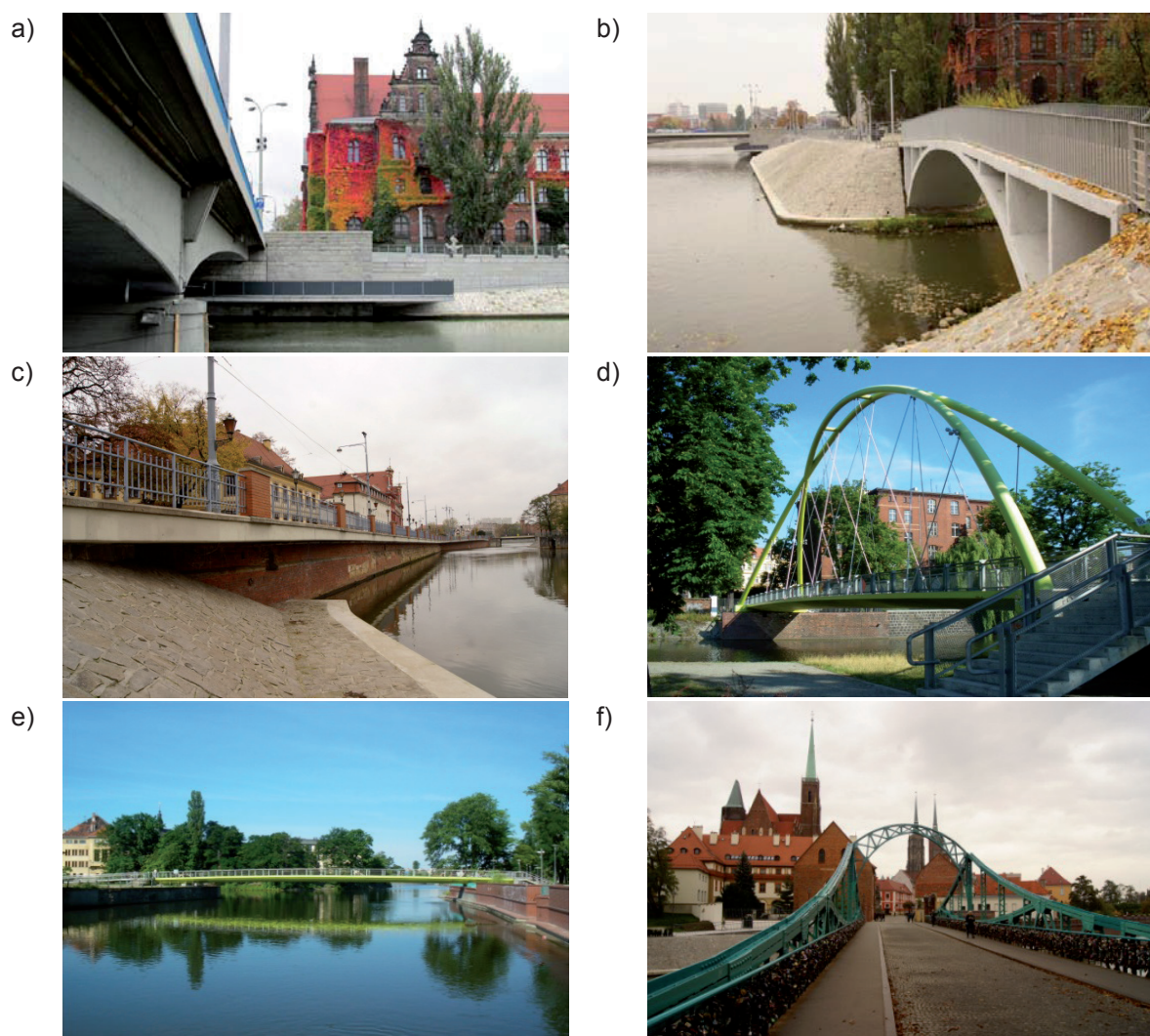
Fig. 1. The main engineering structures along the tourist route developed in the historic centre of Wrocław: a) the deck placed on a cantilever under the Peace Bridge, b) arch footbridge (1928), c) pedestrian route on a cantilever along the embankment of the Odra River, d) Malt Footbridge (2003), f) Tumski Bridge
